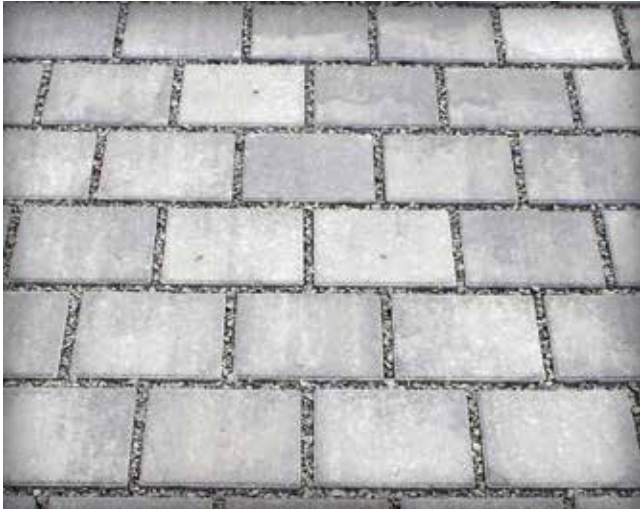
Figure 4. Keeping PICP joints filled with permeable aggregate facilitates removal of accumulated sediment.
