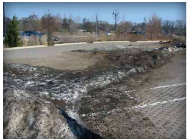
Figure 24. This is an example of snow that should have been deposited on a grassy area. If such areas are not available, then vacuum clean the PICP in the early spring.
