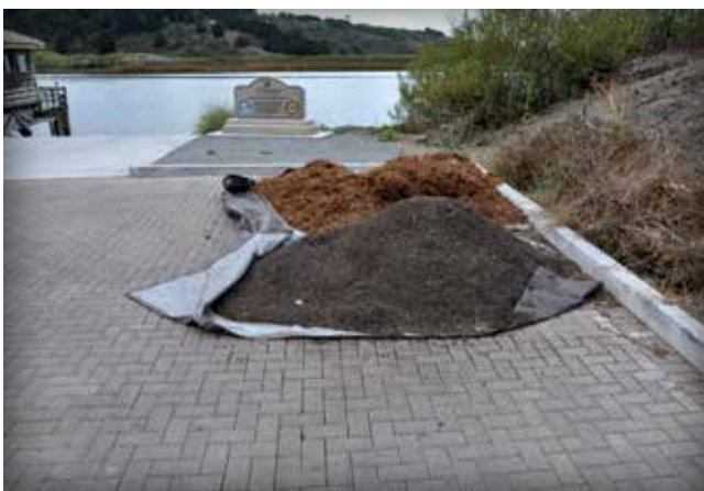
Figure 5. Mulch placed on tarps prevents more expensive cleaning of PICP.
